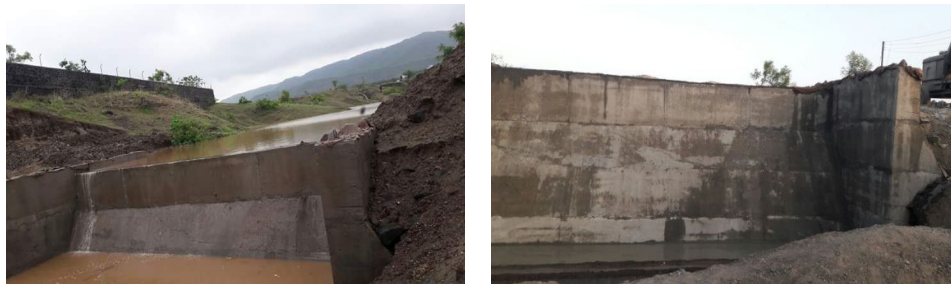
Check dam construction at Satara Village
